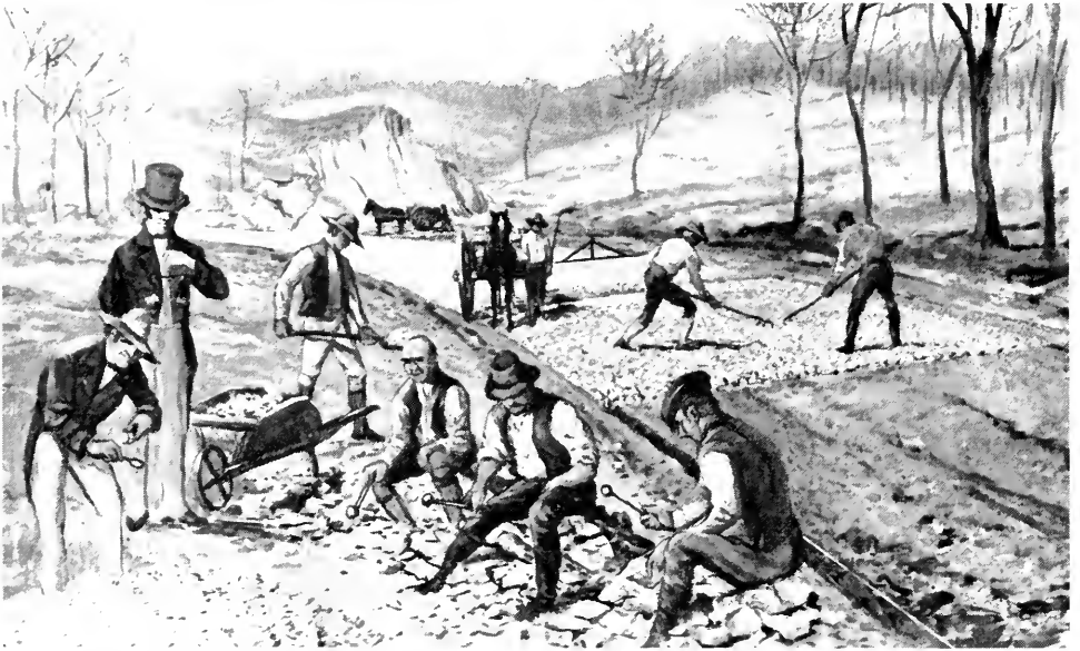
Rebuilding the National Road in 1834. Workmen sit on the ground breaking stone with a small hammer. The inspector at left is testing the stone to see if it will pass through a 3-inch ring. The one next to him is weighing each stone to keep it down to 4 ounces. At right laborers spread the fine stone on the prepared roadbed with horse rakes. The surface was rolled smooth and compacted by the traffic that used it. The steam roller had not been invented.
